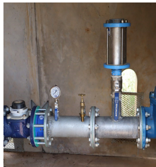
Mokopane Ground Water Refurbishment
