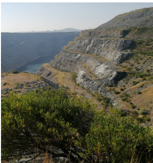
Mogalakwena Mine: Pumping Infrastructure
